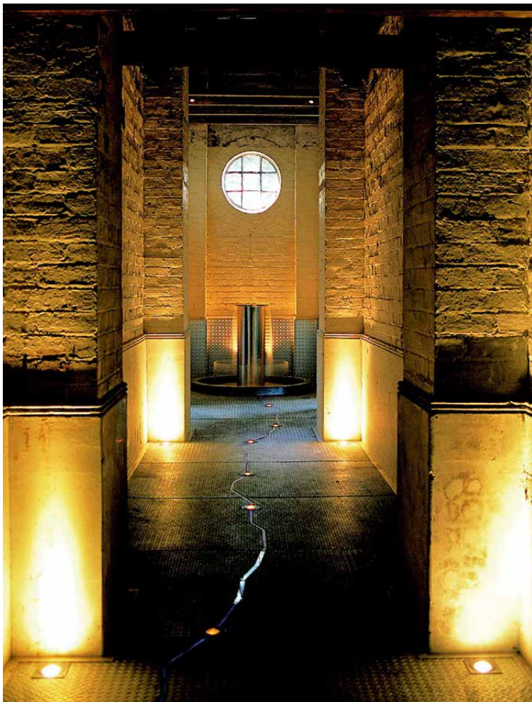
ABOVE: Inside No 1 Pump Station. NTWA
